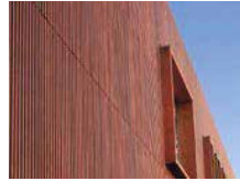
Tianjin Eco City-Jinlu
